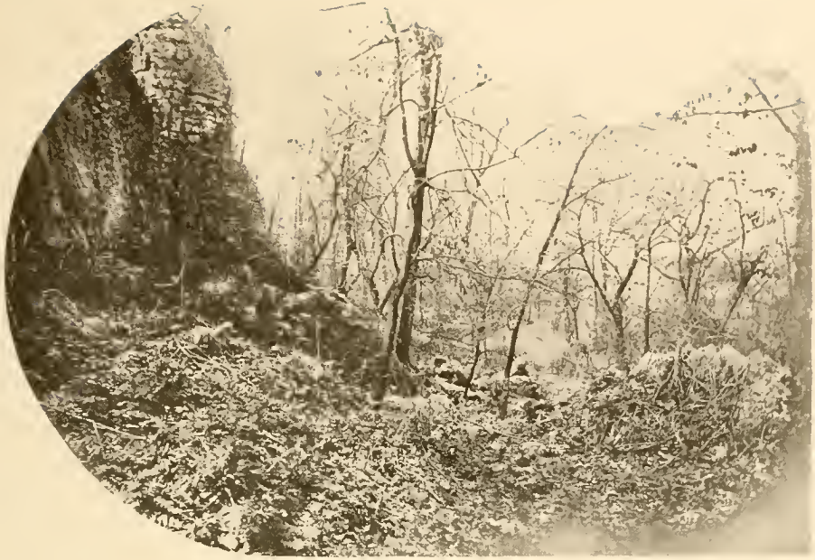
VIEW ON NORTH CLIFF DRIVE BEFORE CONSTRUCTION WORK.
